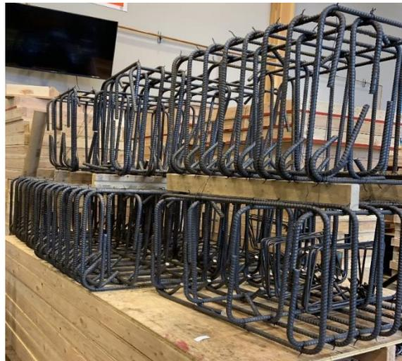
Figure 4.6. Reinforcement Cages for Top and Bottom Blocks
