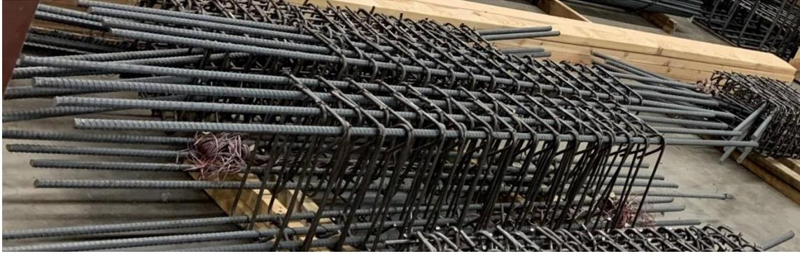
Figure 4.7. Reinforcement Cages for C(#5)-3.0-0.69 and C(#5)-3.0-0.35
