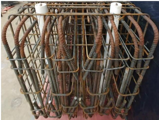
Figure 27 – Reinforcement in Wall Foundation – Confinement of End Hooks.
