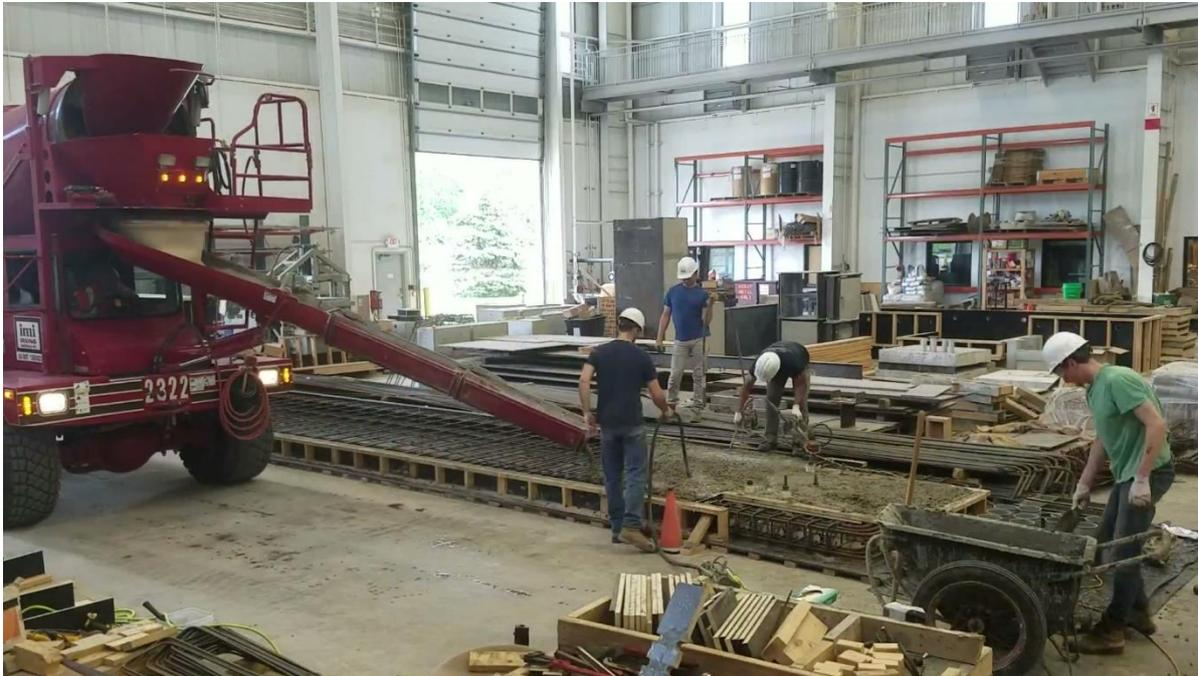
*Figure 42 – First Stage of Casting of Test Wall.*
