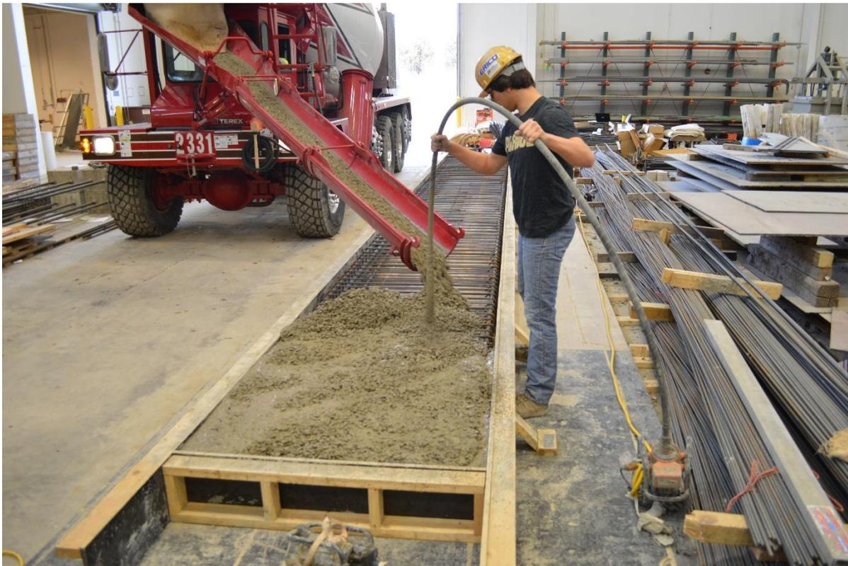
Figure 38 – Casting of Test Beam.
