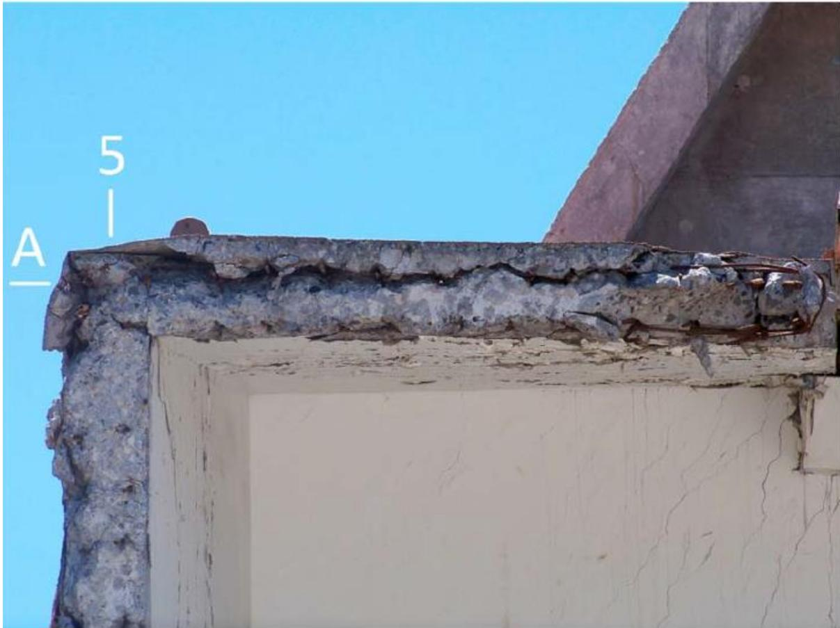
*Figure 2 – Longitudinal splitting observed in Concepcion, Chile, Alto Rio Building, 2010 (Song, 2013).*
