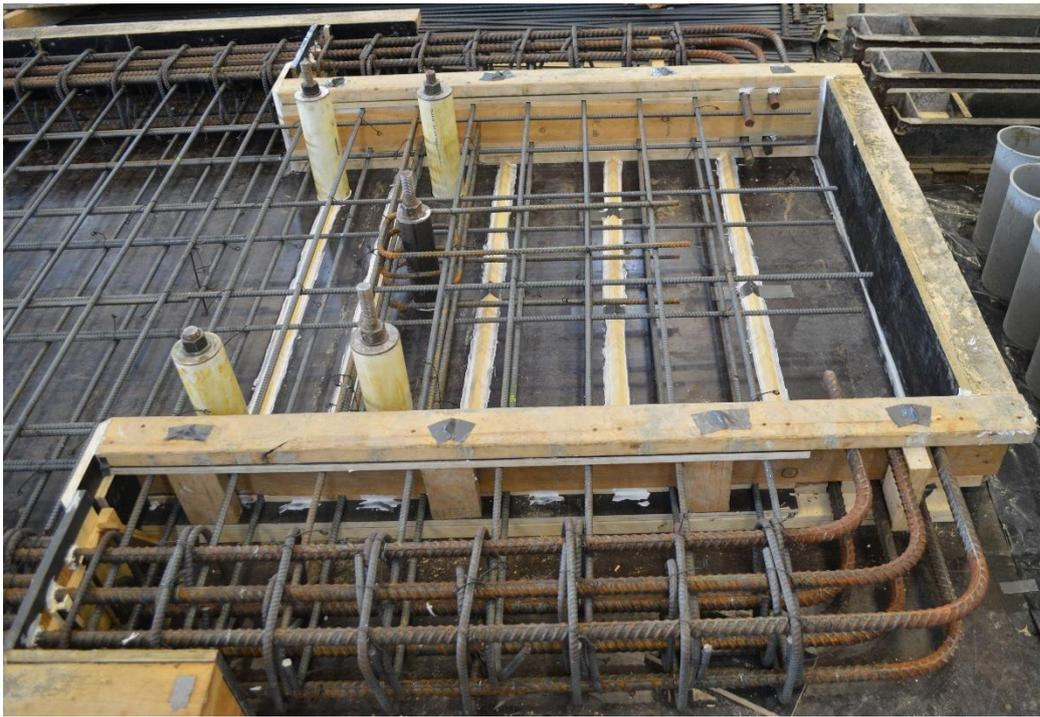
*Figure 43 – Photographs of formwork built around spliced reinforcement near base of test wall.*
