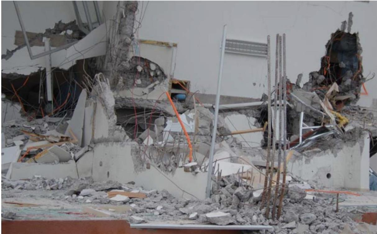
*Figure 4 – Failure of lap splices reported by Song (2013).*
