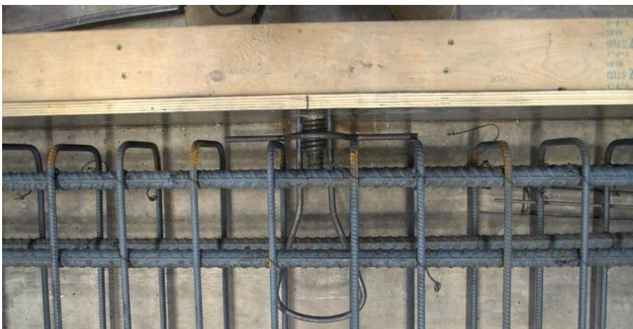
Figure 39 – Lifting Inserts used in Test Beams.
