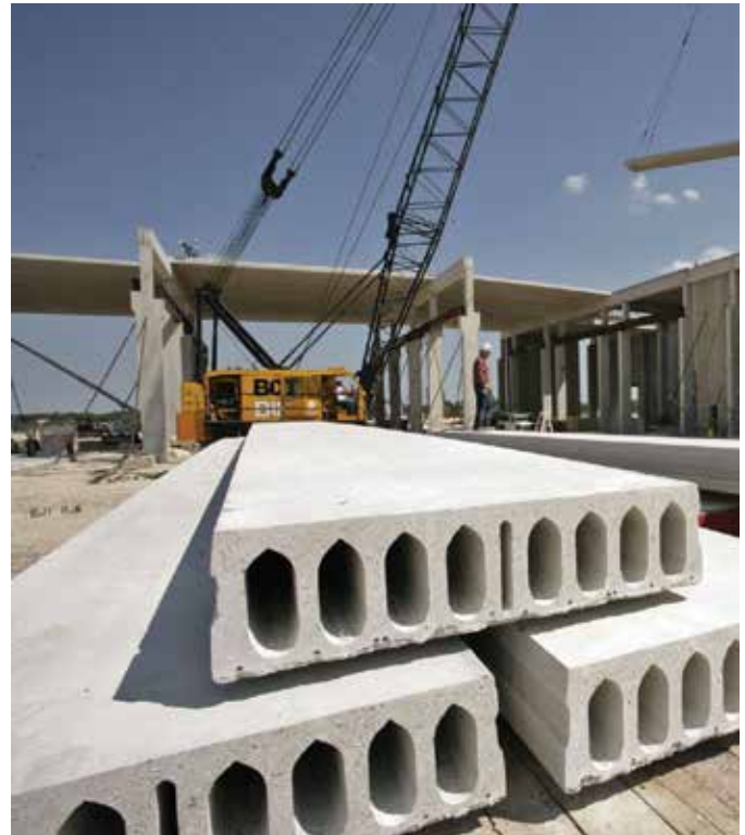
Hollow-core slab installation (photo courtesy of Spancrete, Waukesha, WI)
