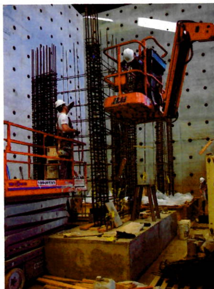
Reinforcing bar assembly, first lift, for research project "High-Strength Steel Bars in Earthquake-Resistant T-Shaped Concrete Walls" (photo courtesy of Andrés Lepage)
