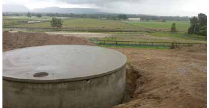
Installation of a concrete water tank
