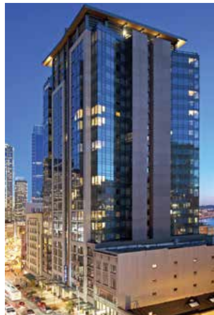
Victoria Apartments, a 24-story residential tower in Seattle, WA
