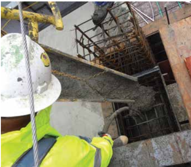
Casting a fiber-reinforced concrete coupling beam
