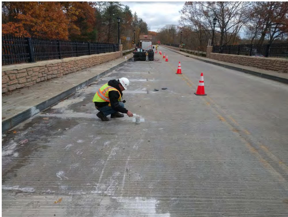
Fig. 17–Coring operation of Cuyahoga Bridge
