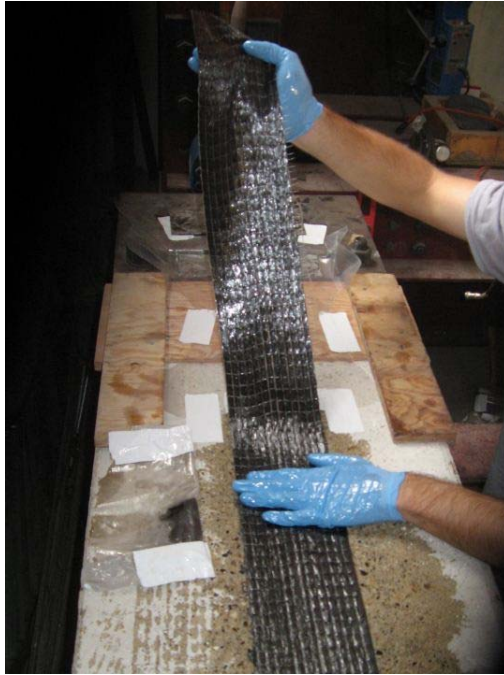
Figure 3.11 FRP sheet is laid onto concrete surface starting from one end. A paint roller is used to eliminate trapped air. A second layer of epoxy is applied to the sheet.
