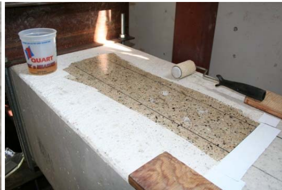
Figure 3.8 FRP anchors are trimmed, prior to applying epoxy, to ensure correct splay diameters
