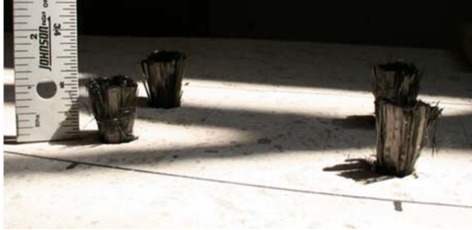
Figure 3.8 FRP anchors are trimmed, prior to applying epoxy, to ensure correct splay diameters
