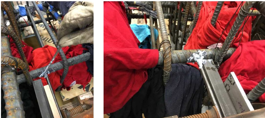
Figure A-15: Brass-Brazing Procedure - Step 2: Application of Heating Chemical
