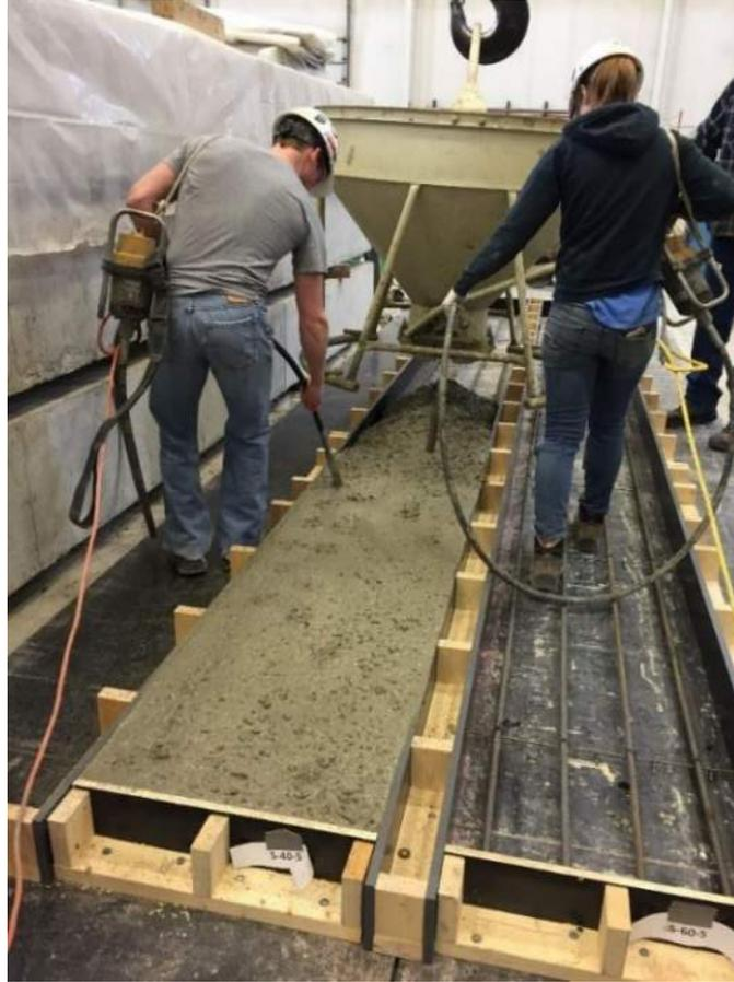
**Figure 3.16: Series V Consolidation Process**
