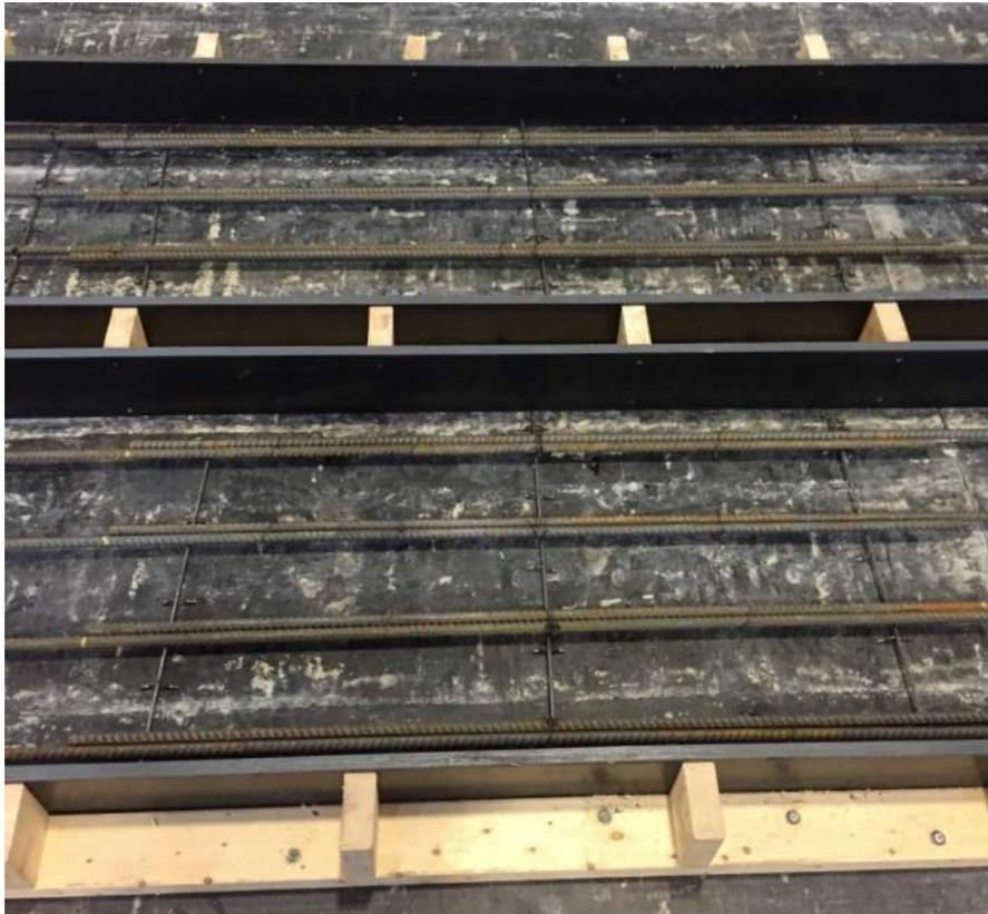
**Figure 3.13: Slab Construction – Splice Region**
