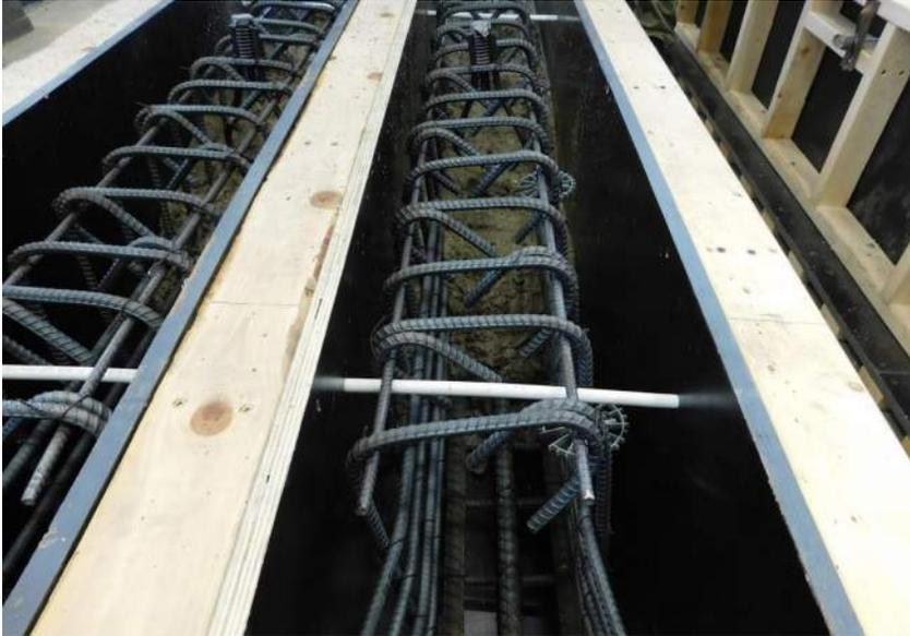
**Figure 2.17: Reinforcing Cages Inside Forms**
