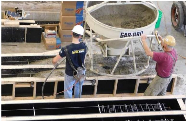
**Figure 2.19: Casting Procedure for Specimens**
