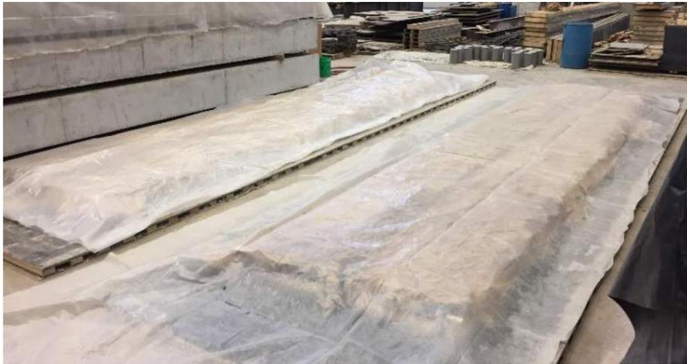
**Figure 3.19: Series V Moist Curing**
