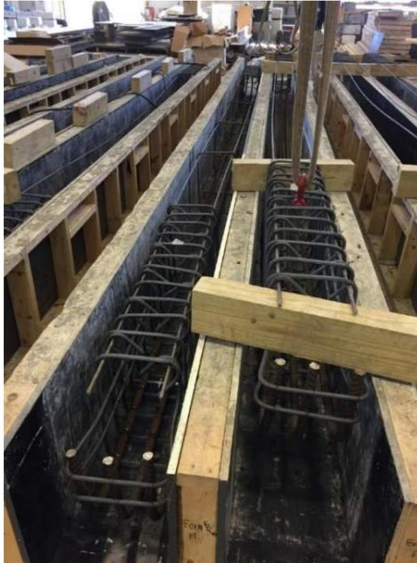
**Figure 4.18: Beam Shear Region and Cage Lifting**
