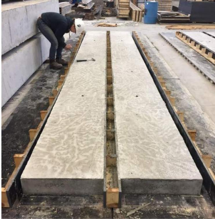
**Figure 3.20: Series V Side Form Removal**
