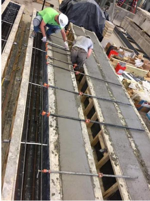
**Figure 4.23: Series VI Form Bracing**
