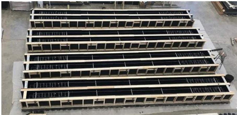
**Figure 2.16: Completed Formwork**
