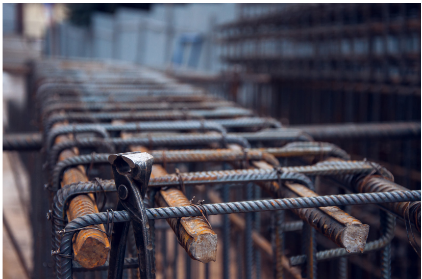
Figure 1.1: Plain steel reinforcement prior to concrete placement. If reinforcement is required, corrosion resistance and structural requirements contribute to the long-term durability of concrete construction.
