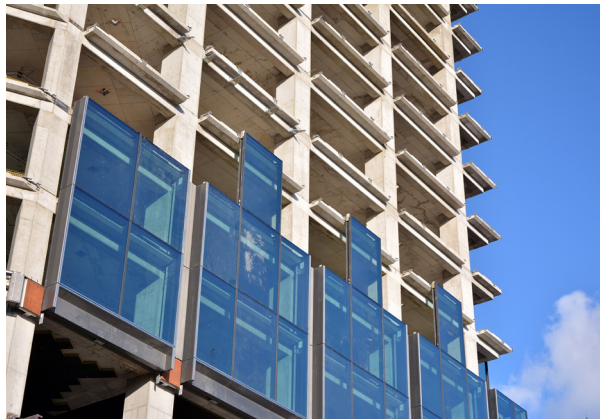
Figure 3.3: Comparison of concrete structures requiring reconciliation of durability design requirements with structural requirements. Concrete primary structure that will be protected with a glass facade and protected from the exterior environment (upper left). Boston City Hall constructed with an exposed concrete facade to exterior environment (upper right). Concrete piers exposed to marine environment must be designed to resist these aggressive durability conditions (right).
