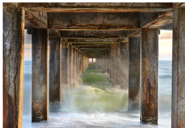
Figure 3.3: Comparison of concrete structures requiring reconciliation of durability design requirements with structural requirements. Concrete primary structure that will be protected with a glass facade and protected from the exterior environment (upper left). Boston City Hall constructed with an exposed concrete facade to exterior environment (upper right). Concrete piers exposed to marine environment must be designed to resist these aggressive durability conditions (right).
