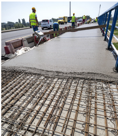
Figure 1.2 Sequence of concrete batching (top), testing (middle), and placement (bottom). Verification that durability design requirements are met through construction is essential.
